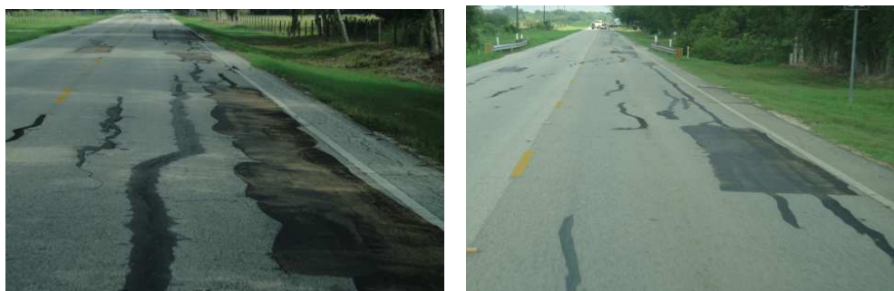
(a). Typical Condition of FM 1887 (SB)
